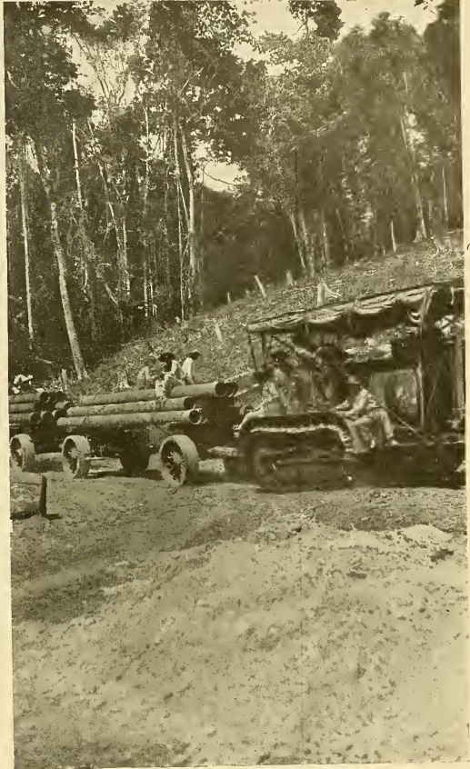
HAULING THE PIPES
